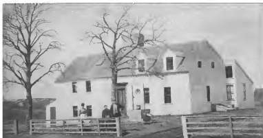
The Hart house about 1890. The room currently installed in the Museum was on the first floor, to the left of the door. When it was built, the house consisted of only the left half of the structure in this photograph and did not include the small lean-to.
